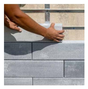
The U-Cara Wall Mount System allows you to put the finishing touches on your project by cladding existing structures
