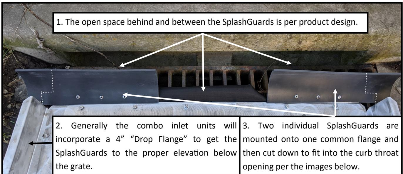
The image and notes above reinforce the basic look and concept of the dual SplashGuard flange associated with ScreenBox installations in combination (curb throat) inlets.
