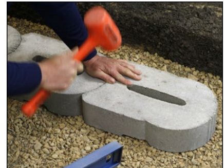
Diagram 3—Lay and level base block
