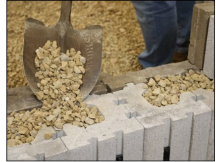
Diagram 5—Fill cores with free draining aggregate
