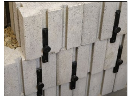
Diagram 6—Lock connector to the block in front
