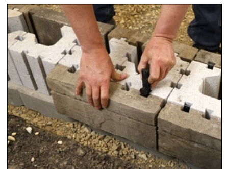
Diagram 20—Placing veneers onto modular block
