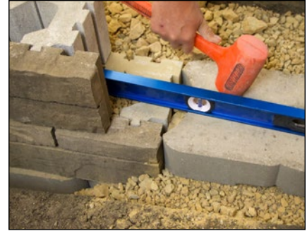
Diagram 7—Stepping up the base
