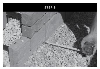
Place 12" of 3/4" drainage rock behind the rear panel of the wall. This will provide for proper drainage behind retaining walls.
