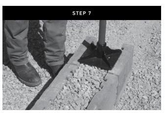
Lightly hand compact the gravel in between the panels for proper compaction.
