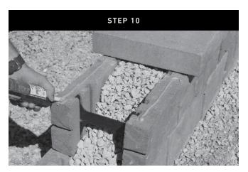
When placing the cap on top of Tandem Wall, use a construction adhesive to secure the cap to the top of the wall.
