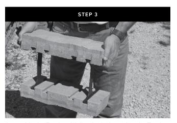
Assemble the Tandem Wall units by inserting the Tandem Wall connectors into the dove tails. Make sure the front and rear panels are the same length.
