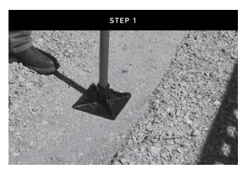
Remove all surface vegetation and debris. Select the length of the wall and excavate a trench the length of the wall and approximately 12" from top of final grade. Then place a minimum of 6" of dense graded aggregate and compact to 95% standard density or modified. It's not recommended to use a pea rock or a rounded type of material on the base.
