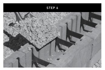
Place 3/4" crushed rock in between the panels to provide frictional connection and proper internal drainage.
