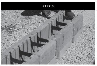
Once the Tandem Wall units have been placed. Run a string line along the back of the front or rear panel to assure you are keeping the wall units straight in line.
