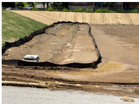
The sides of the basin are covered with erosion control blankets to protect the grass seed as the vegetation is established. The bottom of the basin will be covered in ECBs and vegetated as well.
