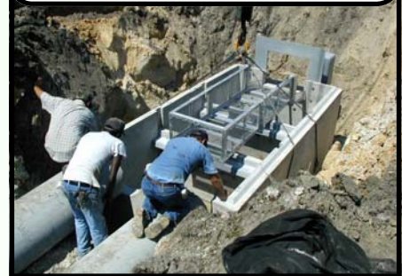
Step 2: Hook up pipes
