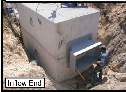
Ready to position inflow pipe and seal pipes with grout
