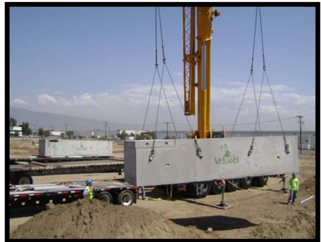
Lifting knuckles and corner protectors must be used to lift the Modular Wetland off the truck.
