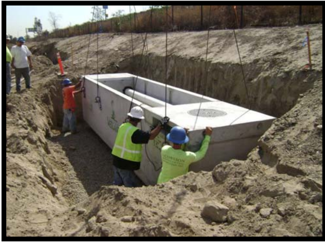
The Modular Wetland is lowered into place.
