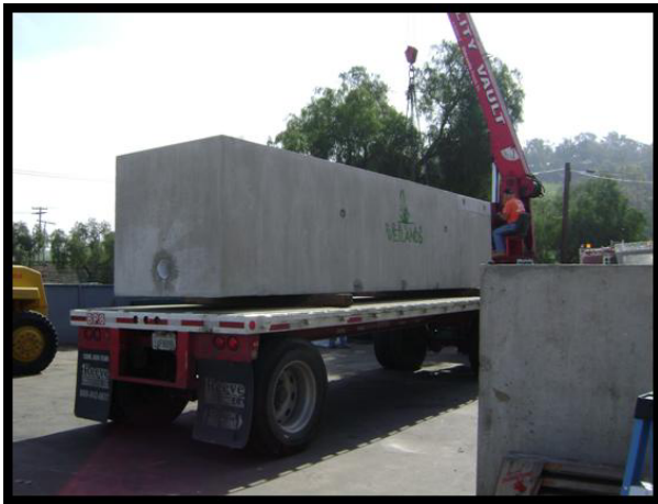
Pre assembled Modular Wetland system loaded at manufacturing plant. Delivery truck is routed to installation site.
