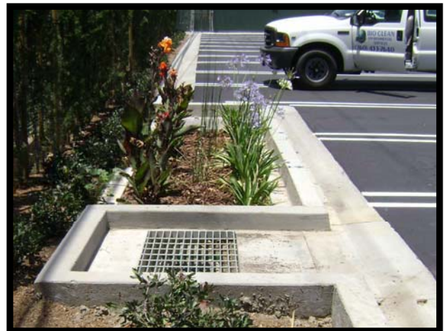
Pavement is pored and vegetation is planted. Once the site is stabilized and cleaned the system is ready to activate.
