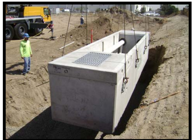
The Modular Wetland is position over the excavation area.
