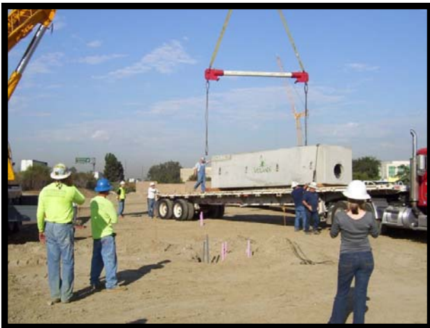
A spreader bar must be used to pick up the Modular Wetland. 8 lifting points (4 on each side) will be provided to lift system.
