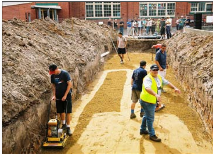
Establish a smooth and level working platform.
