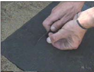
Cut X slightly smaller than pipe as fabric will stretch, making a tighter boot.
