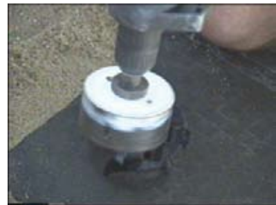
Core drill into the Atlantis matrix plate.
