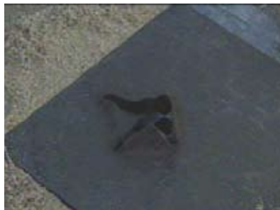
Raised X cut geotextile and liner.
